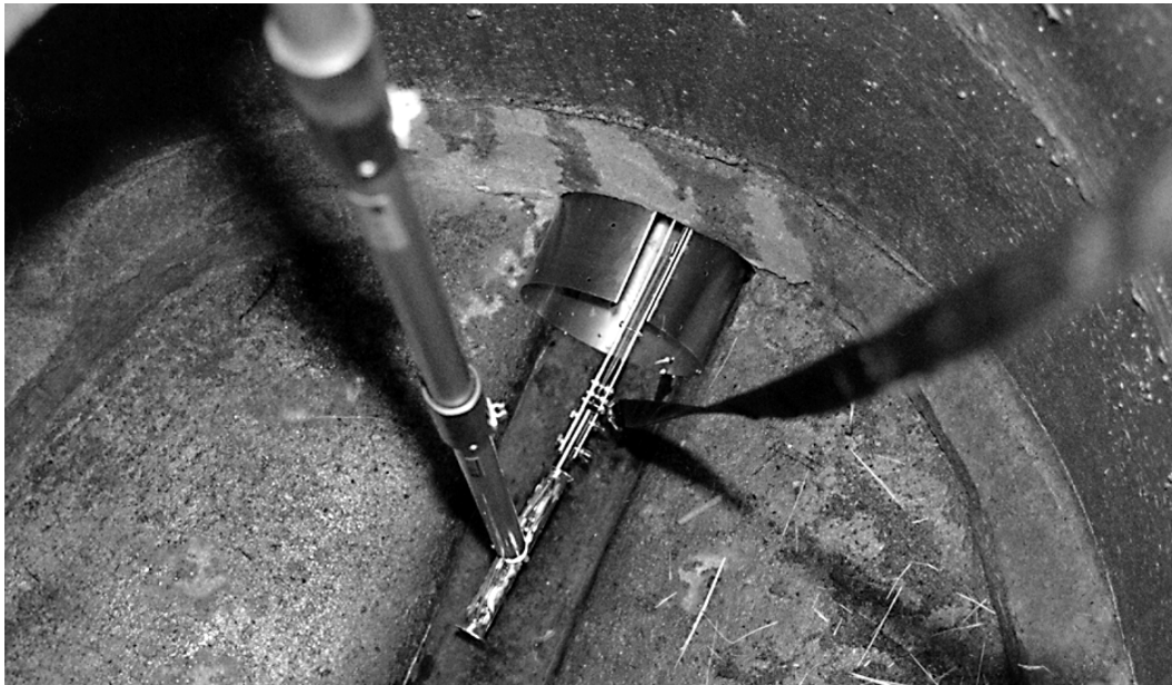
Figure 4-6 Inserting the Ring in the Upstream Channel
